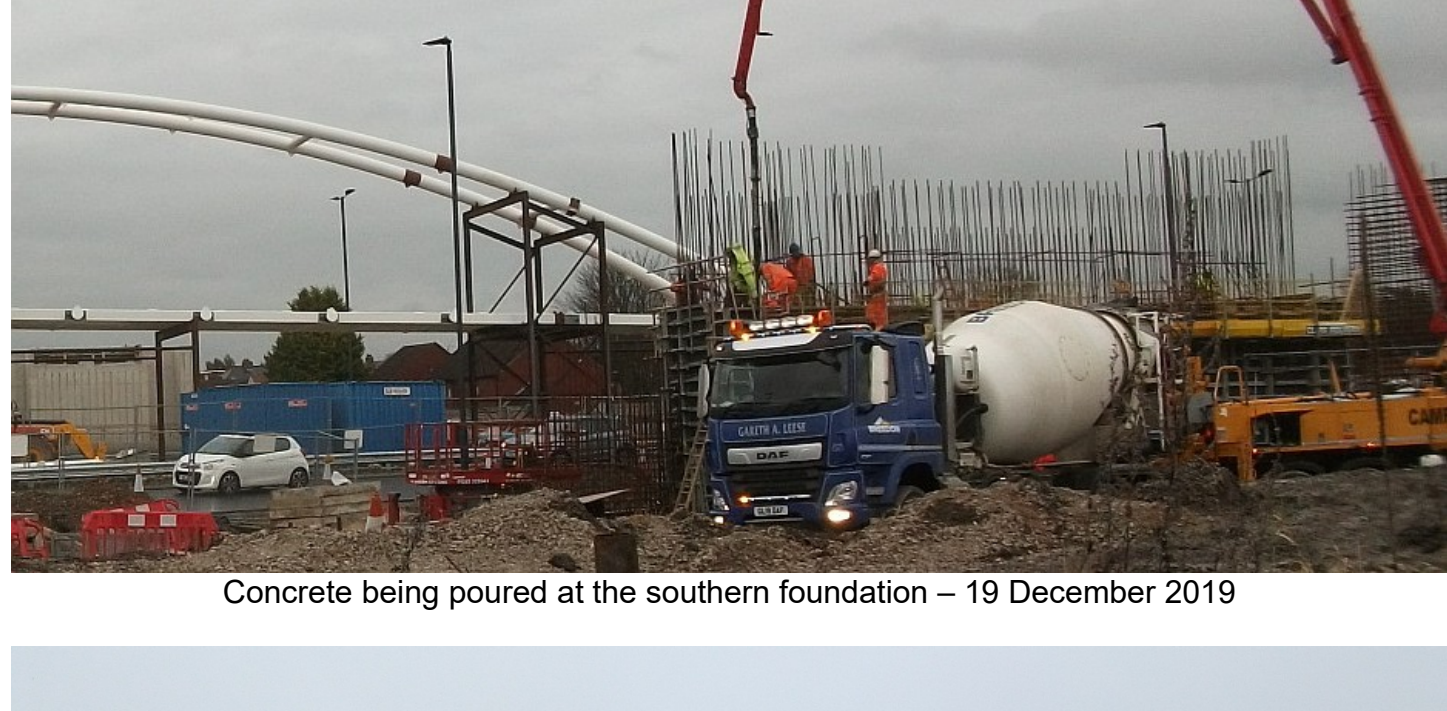
Concrete being poured at the southern foundation – 19 December 2019
