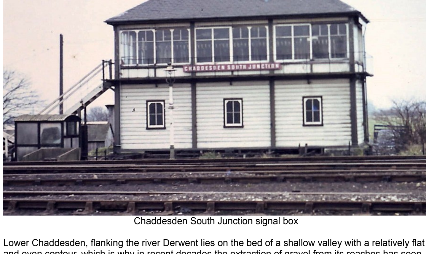
Chaddesden South Junction signal box
