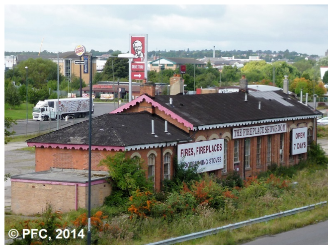
Fig. 12: The remaining northern part of the Wagon Repair Workshop, demolished in 2021.
