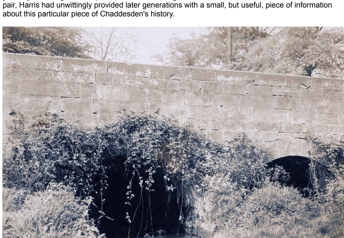
Fig. 4: Bridge adjacent to the sheepwash, Nottingham Road, Chaddesden.
