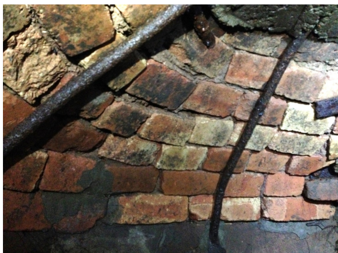
Fig. 3: The chamber roof. Note how the topmost courses of bricks are corbelled inwards and the metal supporting ribs.
