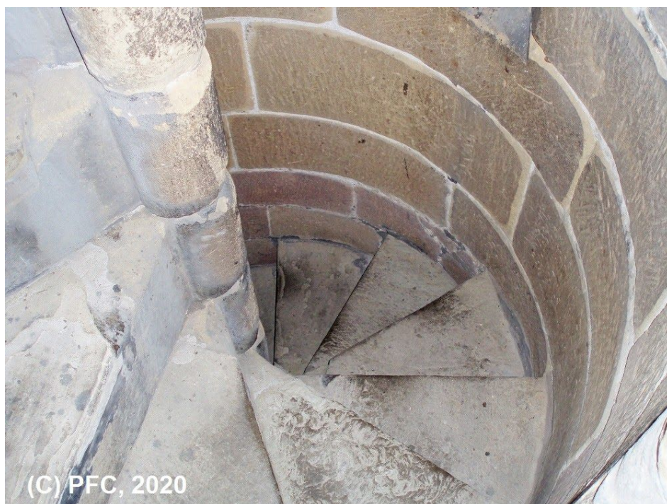
Fig. 3: Looking down the spiral staircase
