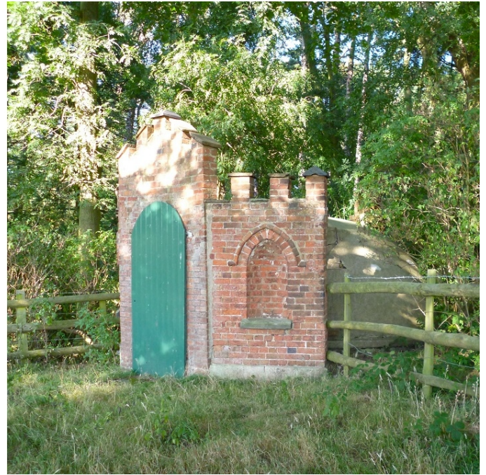
Two views of the ice-house at Locko Park taken in August 2015. Note the exposed and rendered dome of the ice-well visible in the second picture. © Peter Cholerton, 2025
