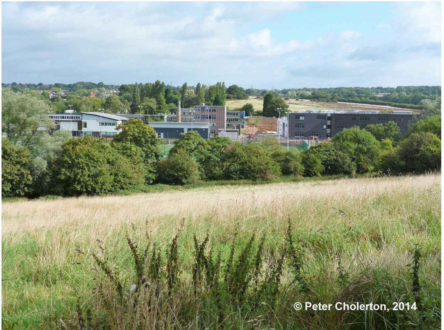
Fig. 7: Pictured here in August 2014, building work at Lees Brook School was well under way close to the actual brook itself (marked by the trees running from left–right) and the site of Bradcar Watermill. In the foreground, land to the north of Windmill Hill is likely to be developed for housing fairly soon.
